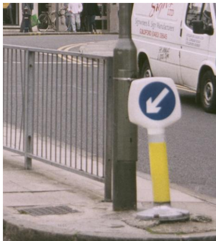
Unnecessary keep left sign and guard rails
