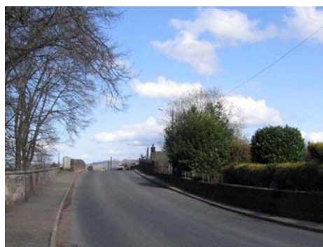
Clifton, hump back bridge after safety scheme
