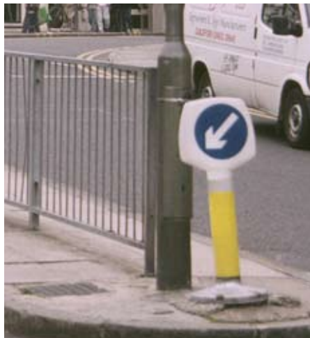
Unnecessary guard rails and Keep left sign
