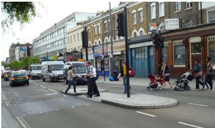
The 1997 pelican crossing regulations allow the option of not installing Keep left signs
